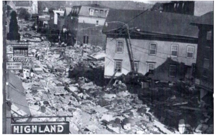
Main Street looking past the end of Elm Street toward St. Joseph Church.
