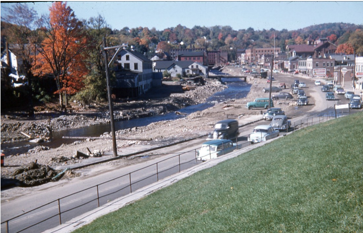
A view of Main Street after demolition of the ruined buildings and before the street was widened
